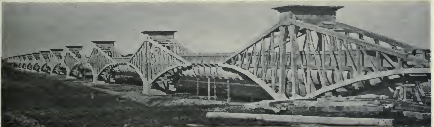
Cantilever Trusses and Cross Beams support oval pipe—Reinforced-concrete construction throughout.
